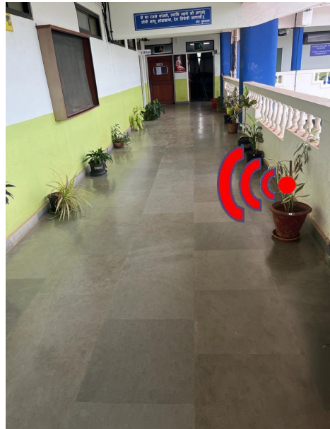
Passages and Hallways
