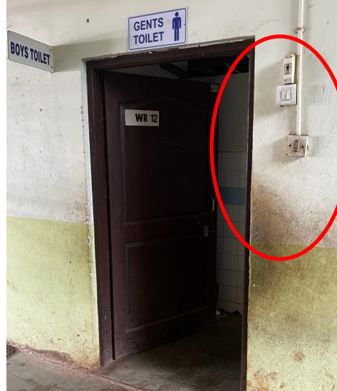
NO COLOUR CONTRAST BETWEEN SWITCHES AND PLATE
