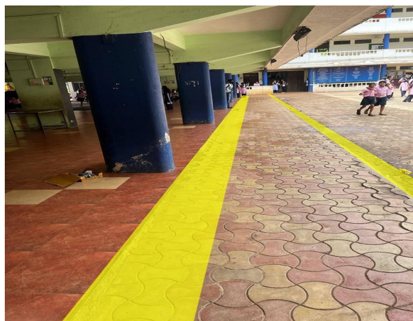
KERBS TO BE PROVIDED ALONG THE SIDE OF THE GROUND AS SHOWN IN THE PICTURE.
