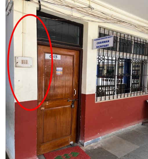
NO COLOUR CONTRAST BETWEEN SWITCHES AND PLATE
