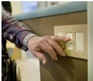
SWITCH BOARD IN CONTRAST WITH THE BACKGROUND
