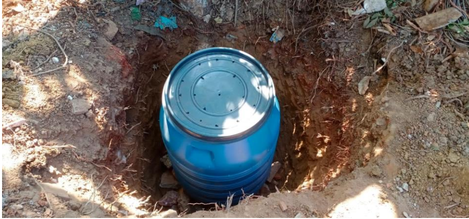
Figure 2: Installation of Tanks
