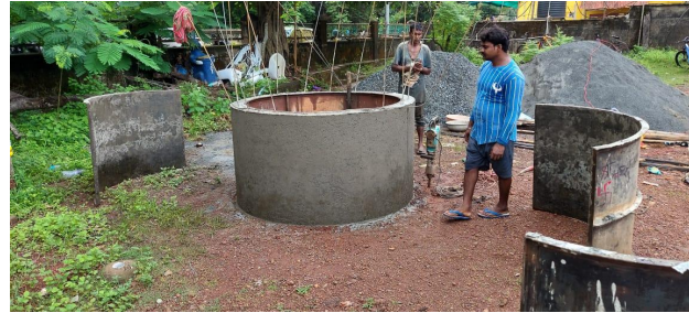
Fig 8: Recharge well ducting construction
