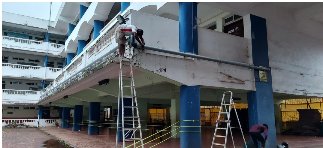
Fig 4: Installation of the plumbing system for rooftop RWH
