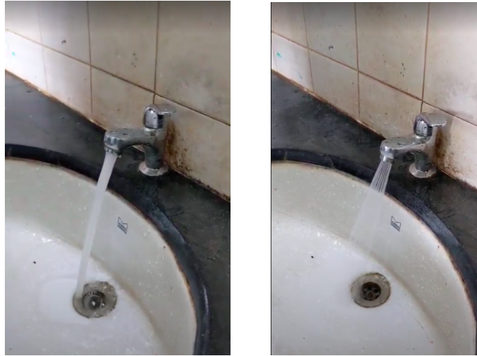
Fig 11: Water flow before(left) & after(right) fixing aerators
