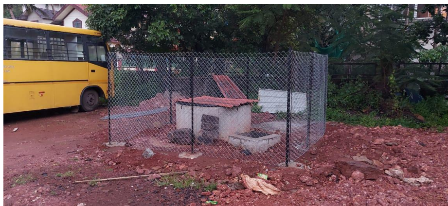
Fig 9: Recharge well protected by safety grill
