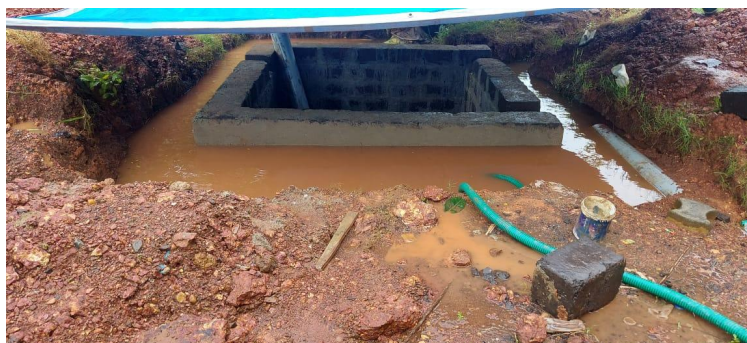
Fig 7: New sump during construction
